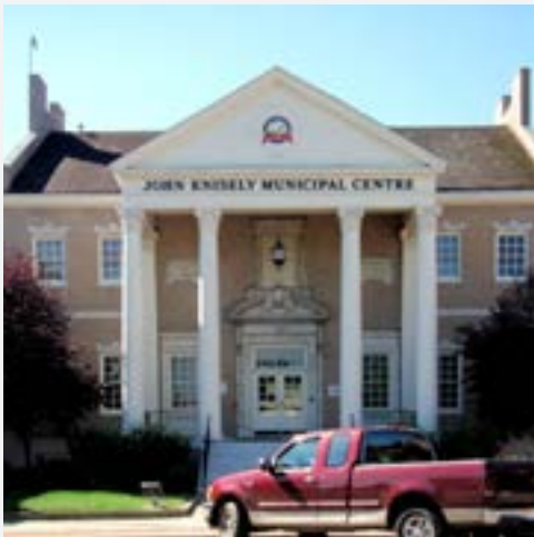
The John Knisely Municipal Centre houses the Mayor's office and City Council.
